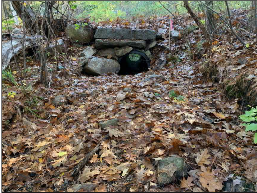
Photograph 1. Essex River, looking south toward culvert below Apple St
