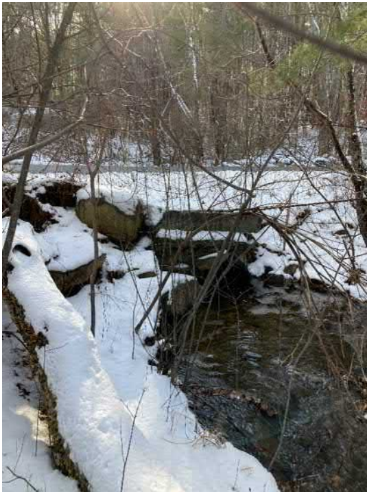
Photo 26 View southerly towards downgradient end of culvert. (1/17/23)
