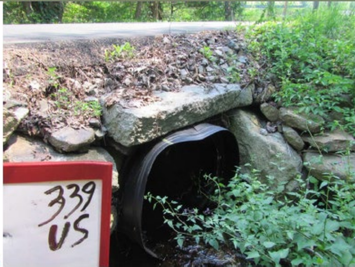
i. Road Over Culvert:
