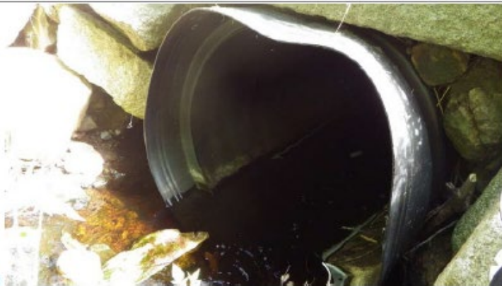
ii. Culvert Inlet:
