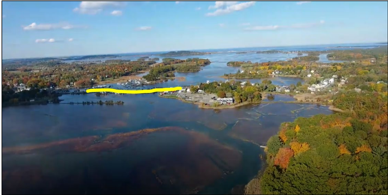
Figure 5. This is an aerial view from the edge of the marsh that abuts Apple Street looking toward the Essex Causeway on Route 133, during a “King Tide”. The Essex River, Essex Bay, and Ipswich Bay are in the distance. The segment of the causeway highlighted in yellow represents the area that typically gets flooded during storm surges and at some astronomically high tides (also see Figure 1). This picture is excerpted from a short drone video shot by DeRosa Environmental in Essex in 2016. You may view the entire video here , which will give you a sense of how Essex is already close to flooding when astronomically high tides are in play. Notice how the entire basin is already flooded well over the top of the marsh platform.
