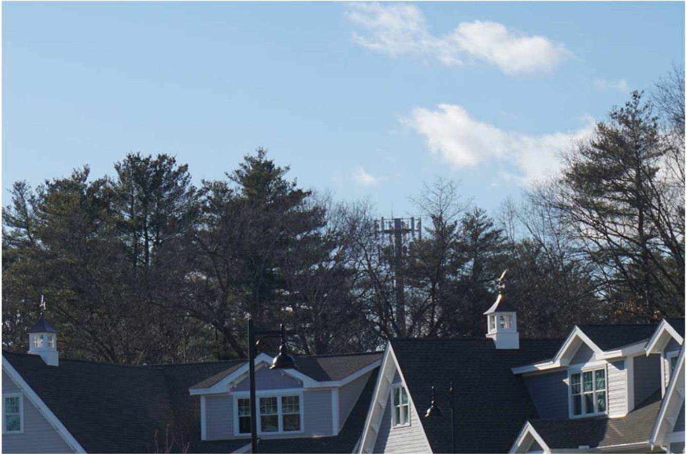
Foreground: Units at the Village at Canter Brook Farm. Background: 120' cell tower
