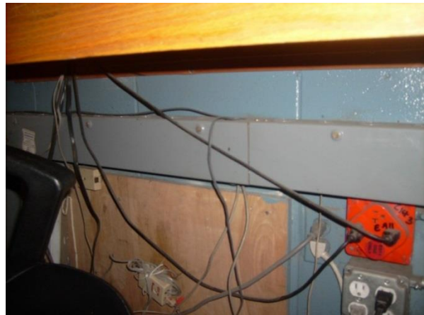
Main Service Entrance and Poor Existing Wiring Standards
