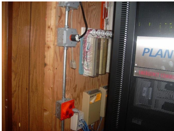
Unprotected Communications Equipment
